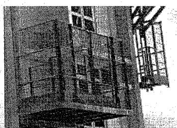
工作平台護欄以金屬絲網圍封。 Parapet wall of a working platform is fenced with wire mesh
